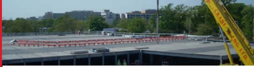
CAR PARK CONSTRUCTION & SAFETY
